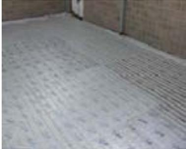
*Hilton Scouts and Guides building, underfloor heating pipe laid on insulating base prior to pouring concrete floor. Pipes at optimal spacing for low temperature heat pump operation.*
