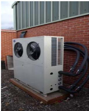
*Hilton Scouts and Guides building, 20kW air source heat pump which provides all space heating and contributes to domestic hot water heating (Picture by David Higgs MBE)*
