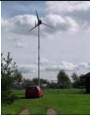
*Manufactured in the East Midlands, Iskra Wind Turbines AT5-1 5kW wind turbine on guyed mast.*
