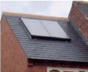
*Flat plate solar collector for water heating installed by T4 Sustainability, "in roof mounting" (flushed into roof)*
