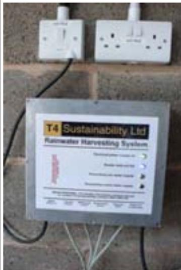
*Hilton Scouts and Guides building, low cost automated controls operate the submersible pump in the underground storage tank, and allow the use of mains water as backup .Picture by David Higgs MBE*
